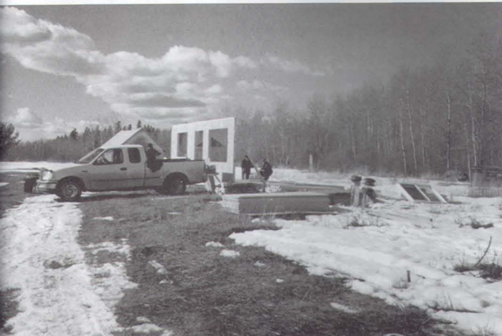
New home construction at Sapwagamik
