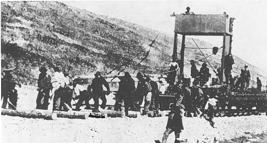
Laying track near Maple Creek: 1883. photo credit: Saskatchewan Archives Board.
