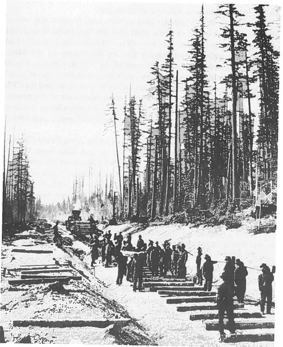
Laying track in the Lower Fraser Valley, 1881
